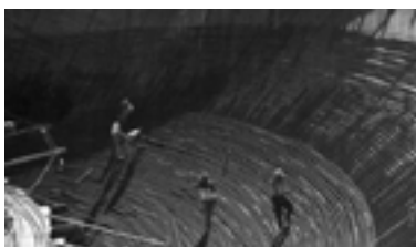
3. The violent labor conditions of Brasilia's building site were part of Sergio Ferro's critique on architectural practice. Image © Marcel Gautherot
