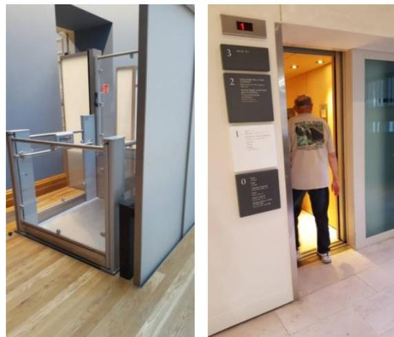
**Fig. 14:** platform lifts or passengers' lifts
